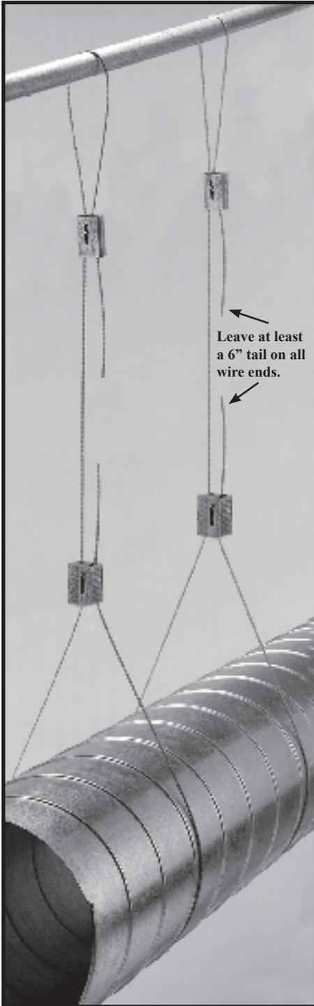
As a matter of sound engineering practice, the Rize Kwik-Loc assembly must be located no closer than 12 inches to the suspension point. In the case of round duct, where the wire rope encircles the duct, the Kwik-Loc must be located the distance of one diameter from the duct wall.
